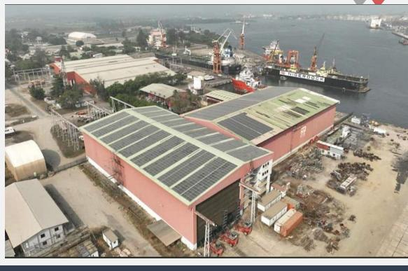
A total of 2360 units of Jinko 545Wp solar panels and 14 units of SMA SHP solar inverters will be installed
